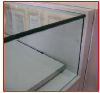
particular of glass top and frontal inside the grooves. please note that glass top lay on glass frontal
